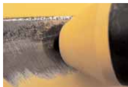
Rust which has penetrated deep inside the metal is removed by blasting.
