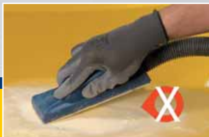
WRONG Incomplete contact between sanding area and substrate.
